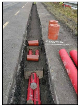
Plate 2-1 110Kv Cable Trench View
