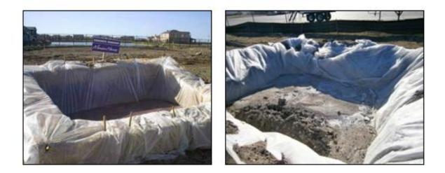
Plate 3-1 Typical concrete wash out areas
